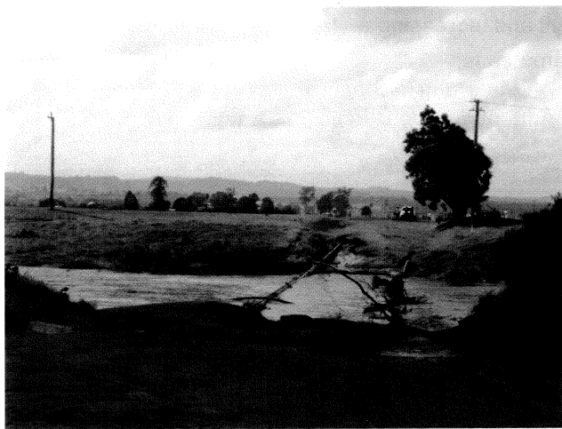
Another bridge downstream of the LVRC Pound
